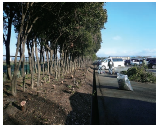
Clearing trees within the plant
