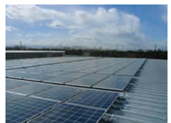
Solar power panels are installed on the roof of our factory
