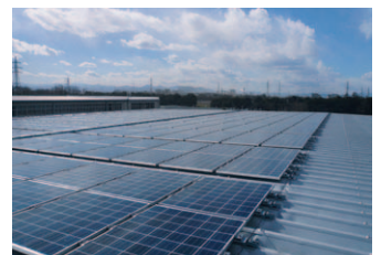
Solar power panels are installed on the roof of our factory
