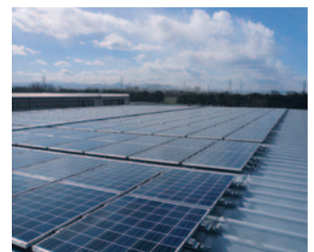
Solar power panels are installed on the roof of our factory
