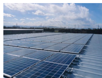
Solar power panels are installed on the roof of our factory
