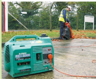
Generator being used for cleaning work
