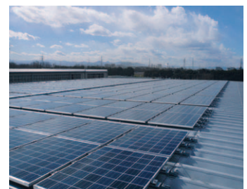
Solar power panels are installed on the roof of our factory
