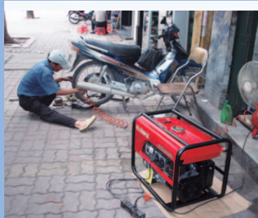
ELEMAX generators actively being used in Vietnam
